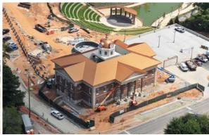
During the last several weeks the final shape of the new City Hall has been revealed. The clock cupola was lifted into position by a huge crane and Mayor Pirkle assisted in installing the spire at the top of the dome. The columns at the entrance were installed and are awaiting paint. The aerial view shows the amphitheater and pond behind.
